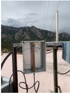
10G antenna with radome removed
